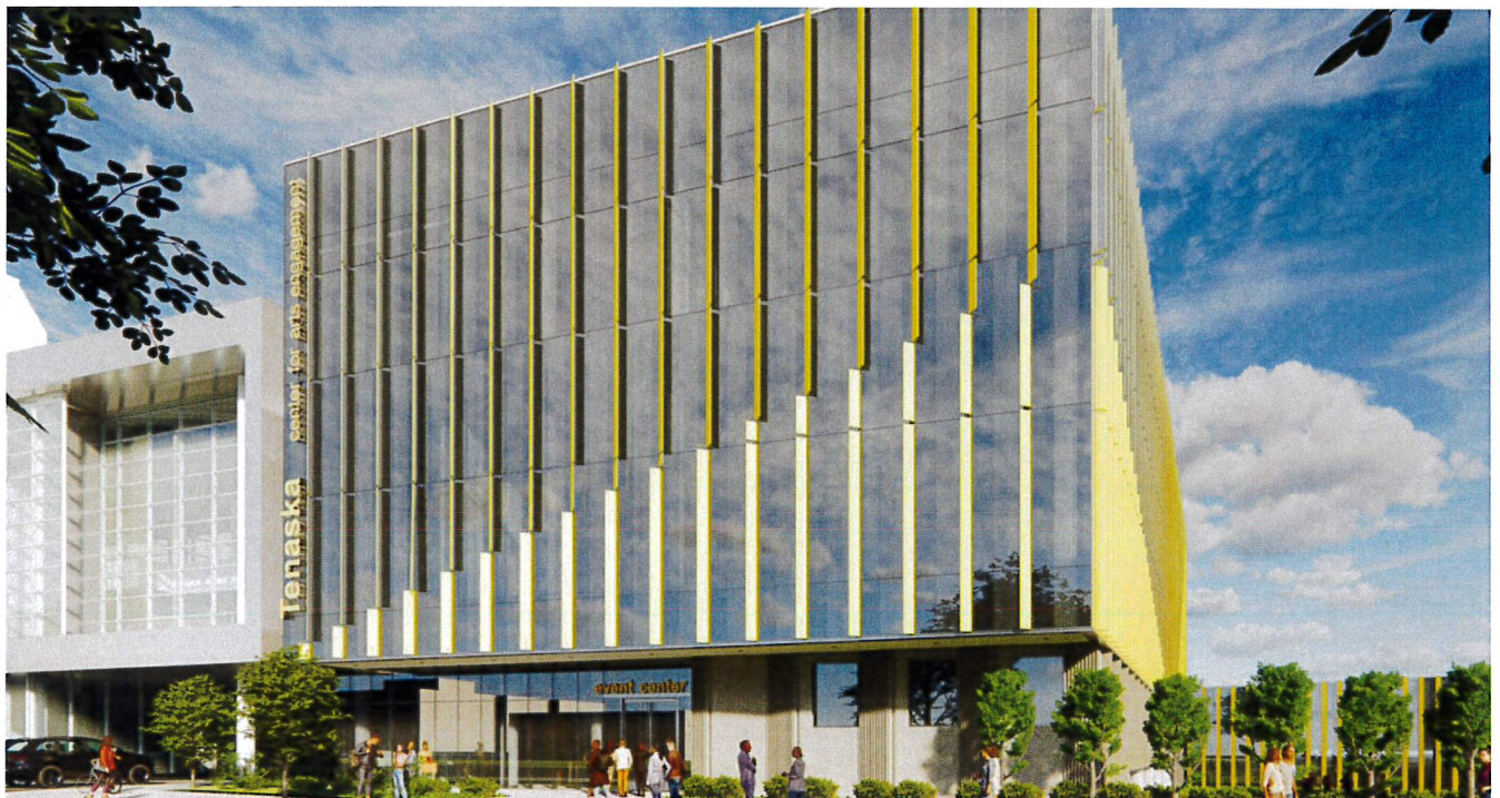
View from Douglas Street, looking northwest
